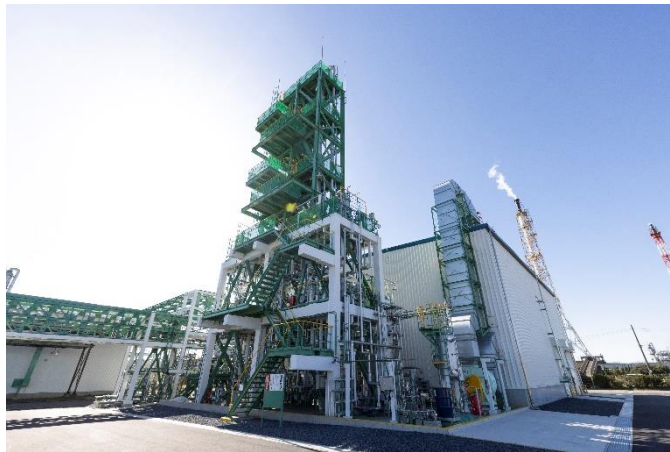
Polystyrene chemical recycling plant
