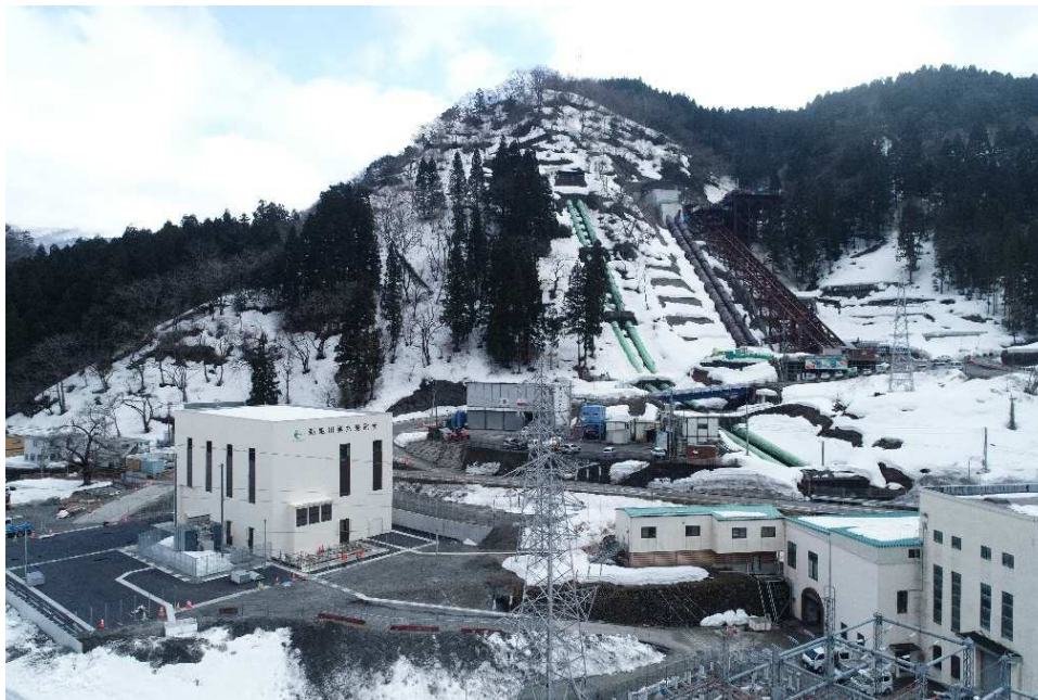
New Himekawa No. 6 Power Plant
