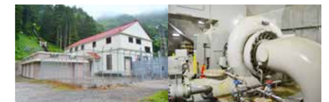
The Kotakigawa Power Plant main building
