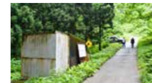
One of the entrances to the tunnel leading to the power plant
