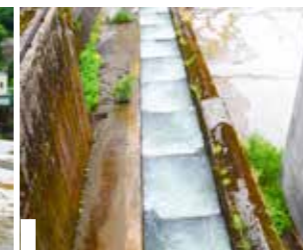
A fishway installed alongside the dam
