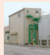
"ER" production plant
