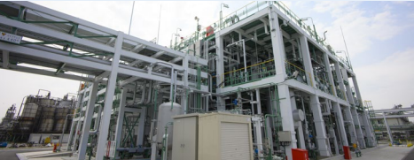
Exterior of the SNECTON manufacturing plant
