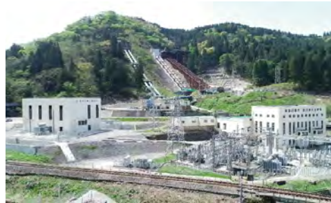
New Himekawa No. 6 Power Plant run by Kurobegawa Electric Power Company which commenced operation in April 2022 (on the left is the New Himekawa No.6 Power Plant, and on the right is the Himekawa No.6 Power Plant).
