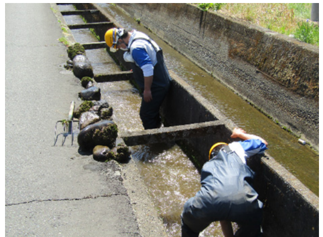
Cleaning of waterway garbage and weeds, and removal of sediment and algae
