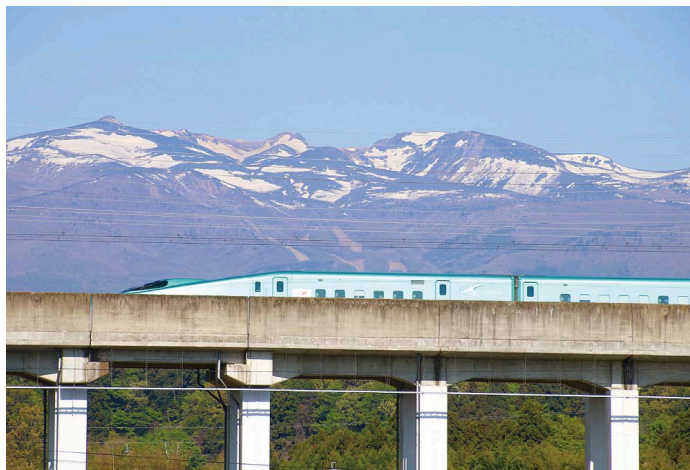
Viaduct of Tohoku Shinkansen (Special admixture, Fukushima Prefecture)
