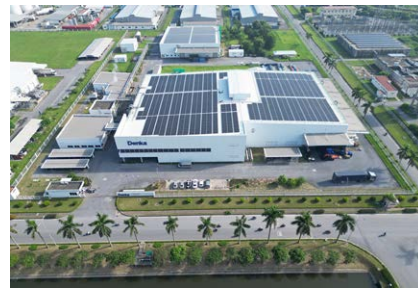
Denka Advanced Materials Vietnam Plant Solar Panels
