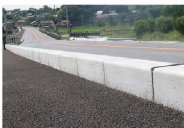
Road boundary block
