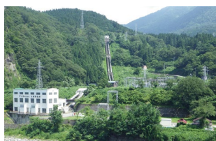
Oami Power Plant (exterior)
