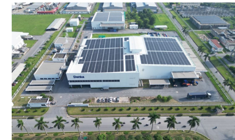
Solar Power Generation PPA at Overseas Site (Vietnam)
