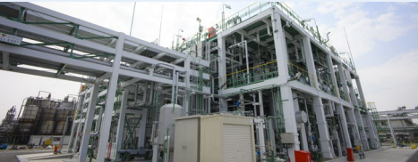
Exterior of the SNECTON manufacturing plant
