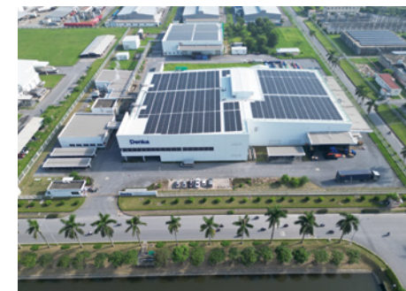
Solar Power Generation PPA at Overseas Site (Vietnam)
