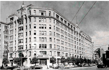
Sanshin Building after construction completed (1930)
