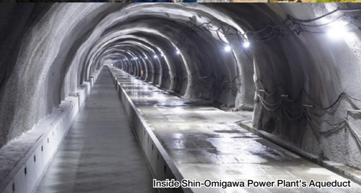
Denka Shin-Omigawa Power Plant
