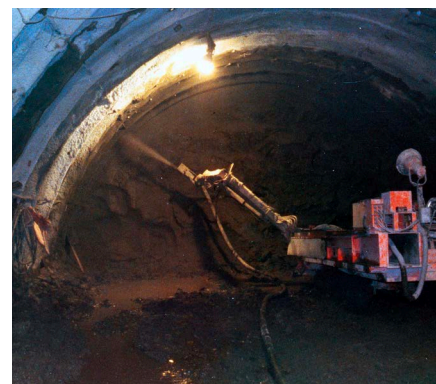
Tunnel spraying work using Denka NATOMIC
