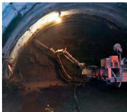
Tunnel spraying work using Denka NATOMIC
