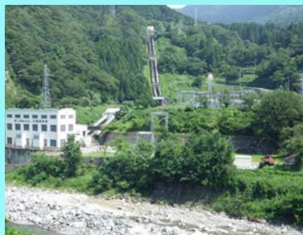
Oami Power Plant
