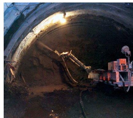
Tunnel spraying work using Denka NATOMIC
