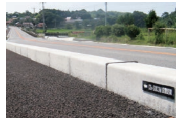
Road curb blocks made using CO 2 -SUICOM (Hamada City, Shimane Prefecture)
