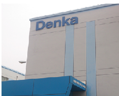
External appearance of DEMDC's new ALSINK plant
