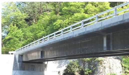
Denka Kotakigawa Bridge
