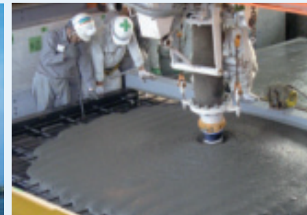
施工例 “SUQCEM” (Super High Quality Cementitious Materials)
