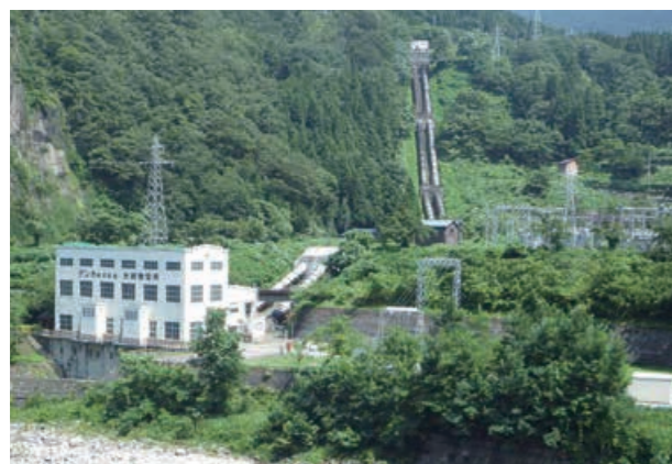
Omi Power Plant concurrently serves as Denka's hydroelectric power generation plant management center
