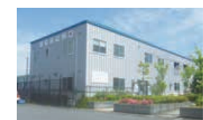
Ekomira Koto processing facility
