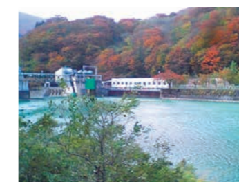
Dam of a hydroelectric power plant
