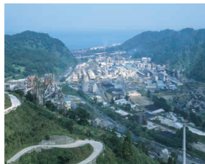
An aerial view of the Omi Plant
