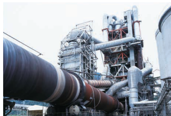
The Omi Plant's cement production facility
