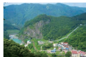
The Oami Power Plant (hydroelectric power generation)
