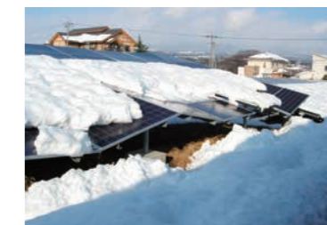
Snow damage at DENKA Solar Power Shibukawa
