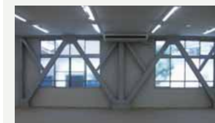
Reinforced wall of the Ofuna Plant's recreation facility
