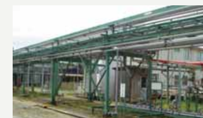
Reinforcing the Chiba Plant's pipe rack modules
