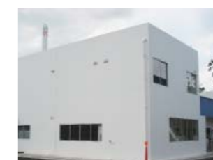
The Technical Service Center
