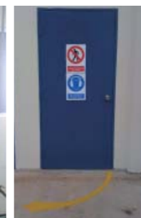
An example of a countermeasure against exposure to a hazard (a cautionary indication is painted on the floor to catch the attention of those who pass by)
