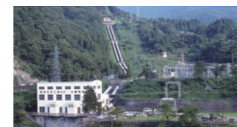
Oami Power Plant
