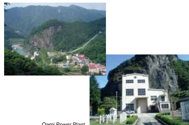
Oami Power Plant
