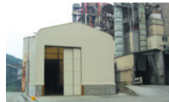
Warehouse to accept sewage sludge
