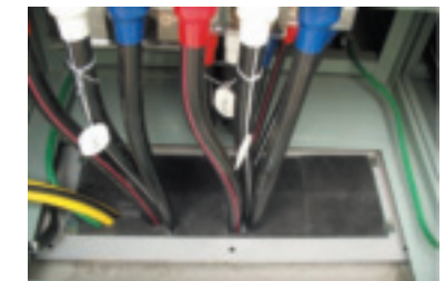
Example of using fire-resistant rubber to prevent conflagration
