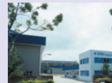
DENKA Advantech/Tuas Plant (Singapore)
