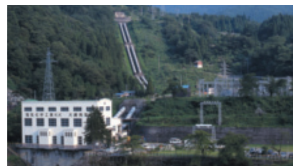
Oami Power Plant
