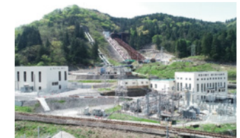
New Himekawa No.6 Hydroelectric Power Plant (started operation in 2022)
