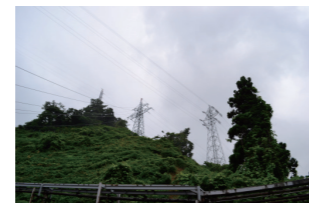
The transmission cables crossing over the mountains distribute electricity from hydroelectric power plants to Denka production facilities
