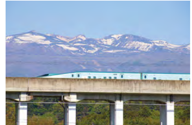
An elevated bridge made using Denka's special cement additives supports the Tohoku Bullet Train Line (Fukushima Prefecture)
