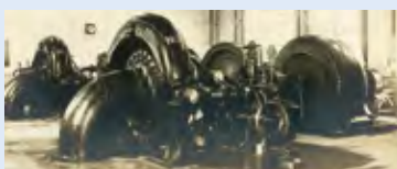
A turbine runner installed in the Kotakigawa Power Plant (photo taken at the completion of the plant)
