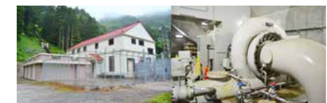
The Kotakigawa Power Plant main building
