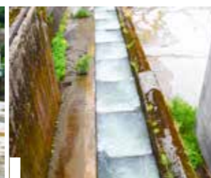
A fishway installed alongside the dam
