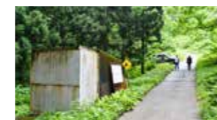
One of the entrances to the tunnel leading to the power plant
