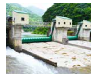
Water intake dam for the Oami Power Plant
