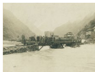
Cover photo The construction of the Otokorogawa Power Plant
