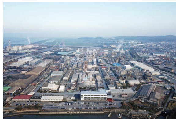
Panoramic view of the Omuta Plant The white building at the front is the Omuta Innovation Hub
