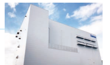
Niigata Plant facility No. 42
