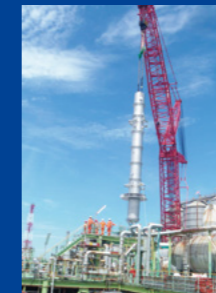
Lifting a new reactor into the air prior to erecting it
