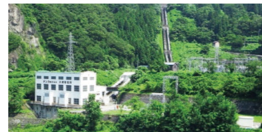
Oami Power Station (Nagano Prefecture)
