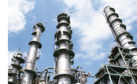
The Styrene Monomer Plant, the largest of our plants in Chiba
