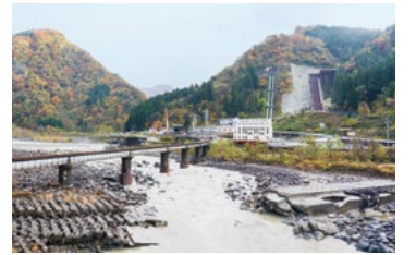
Shin-Himekawa No. 6 Power Station construction site
