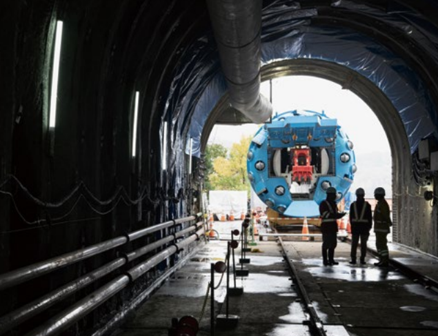
The newly developed NATBM excavator. When it NATM mode, it uses a red bucket tool on the front to safely dig through soft ground.
