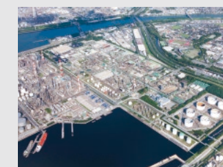
A full view of the Chiba Plant
