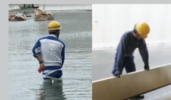
During the flooding, the water was up to our hips (left). Water bars were installed as an emergency measure (right).
