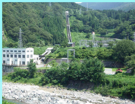
Oami Power Plant
