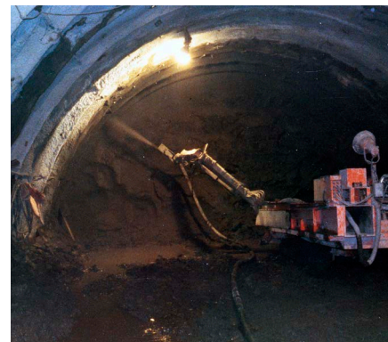
Tunnel spraying work using Denka NATOMIC
