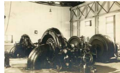
1. A photograph of a Francis turbine runner at Kotakigawa Power Plant (taken shortly after the facility's launch)
