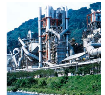
Cement production facility
