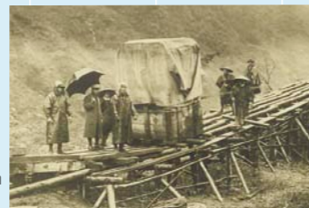
2. A transformer being transported to the under-construction Otokorogawa Power Plant
