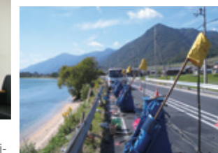
Reinforcing the ground against earthquake damage using DENKA ES
