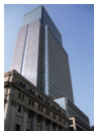
Head Office (Nihonbashi-Mitsui Tower)
