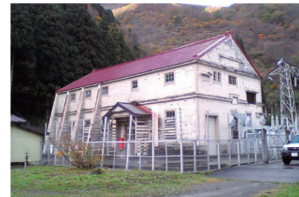
The Kotakigawa Power Plant, operating for 90 years
