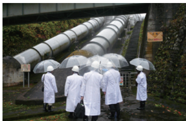
At the Oami Hydroelectric Power Plant
