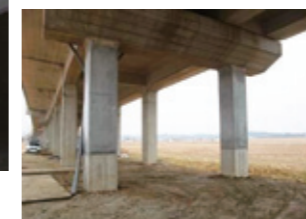
A restored pier
