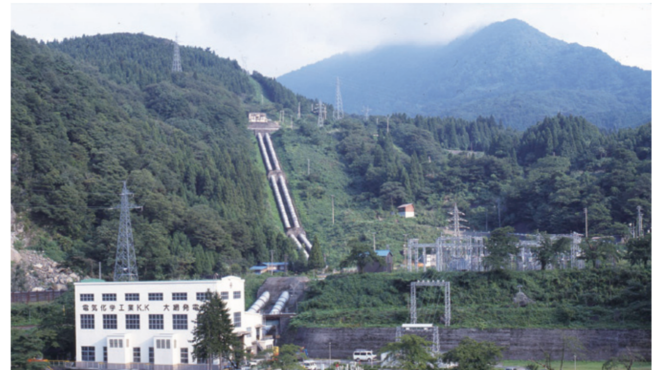
Oami Power Plant
